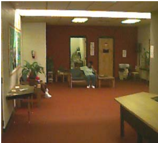
Tired, Worn Carpeting C.W. Griffin Building
