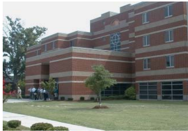
Exterior View, 200-Bed Dormitory
