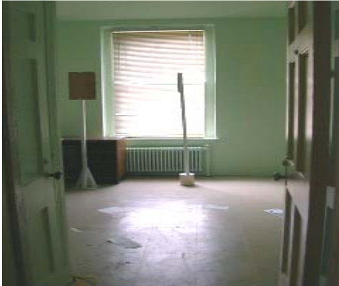
Typical defunct room, Symera Hall
