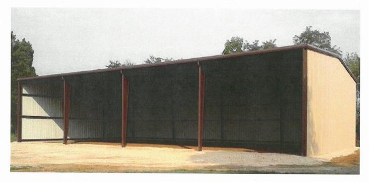
The proposed building is best described as a three-sided, uninsulated, steel framed, steel sided, building with gravel/gravel screenings floor, for equipment storage and maintenance purposes similar in style to the building pictured.
