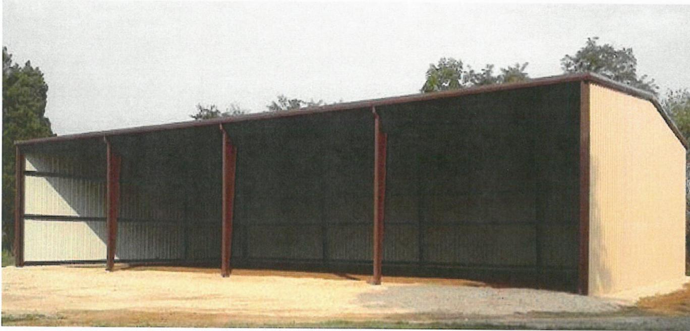
The proposed building is best described as a three-sided, uninsulated, steel framed, steel sided, building with gravel/gravel screenings floor, for equipment storage and maintenance purposes similar in style to the building pictured.
